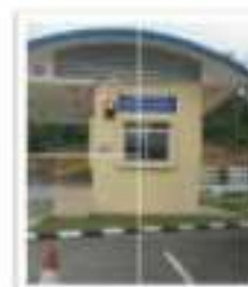
Control Post Inspection Ujong Jalan, Temburong
